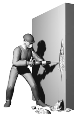
Fig. 2—Bulk concrete removal.
