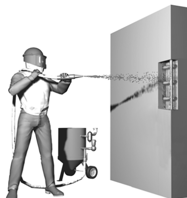
Fig. 4—Final surface cleaning.
