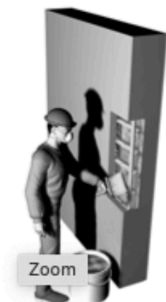
Fig. 6—Treatment of exposed reinforcement.
