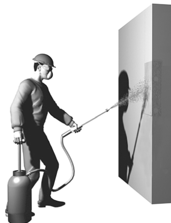
Fig. 9—Spray application of curing compound.
